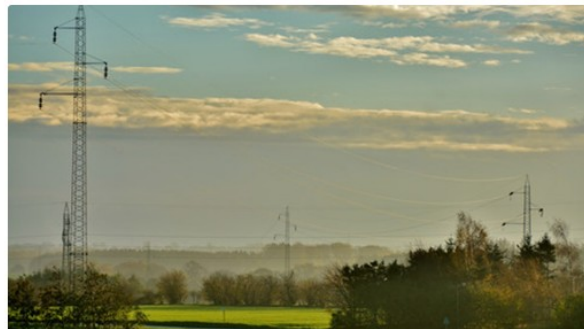
TREFOR Power Grid Living Lab
